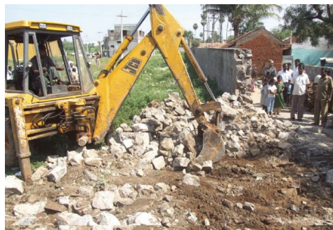
Picture 6.1 Demolition of untouchability wall
